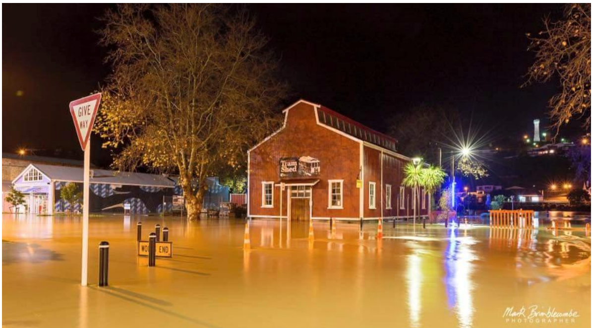
Flood waters surround the Wanganui Tram Shed
